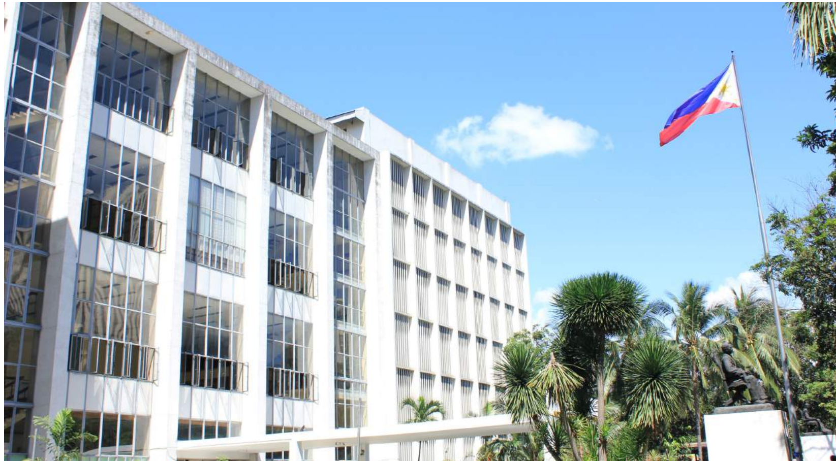
Figure 95. NLP Building in 2011 before the retrofitting and renovation.
