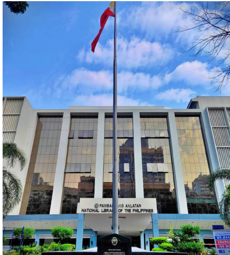
Figures 96 and 97. The present NLP Building after the retrofitting.
